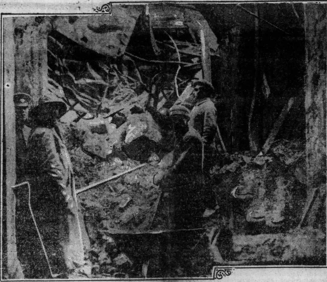
Digging for bodies in the main corridor at the point where the Clock Tower fell in. Here was found the body of Deputy Clerk LaPlante just before the Photograph was taken.
