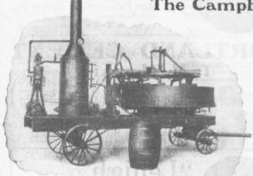
For Mixing Concrete, Cement, Mortar, Plaster and any similar material. The only machine in which material is always in plain sight; that mixes a batch in less than two minutes; that makes a perfect mixture, no matter what class of work is being done.
