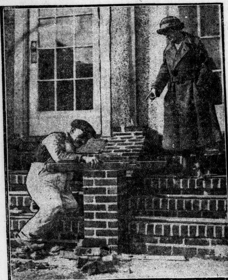
Boss of two hundred men, Miss Wanda Winkill, formerly a nurse, is constructing 54 homes in Maspeth, L.I. A cameraman caught her as she was giving instructions on how to finish a doorstep of one of the new homes
