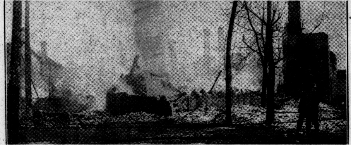
WHERE "FLAMES CAUSED $200,000 LOSS. Ruins of the Grand Shoe Company building after fire early Sunday morning. The scene in Western Ontario in many many factory, Brantford, destroyed fire was one of the most spectacular years.
