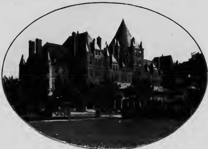
Canadian Pacific Railway Place Viger Station.
