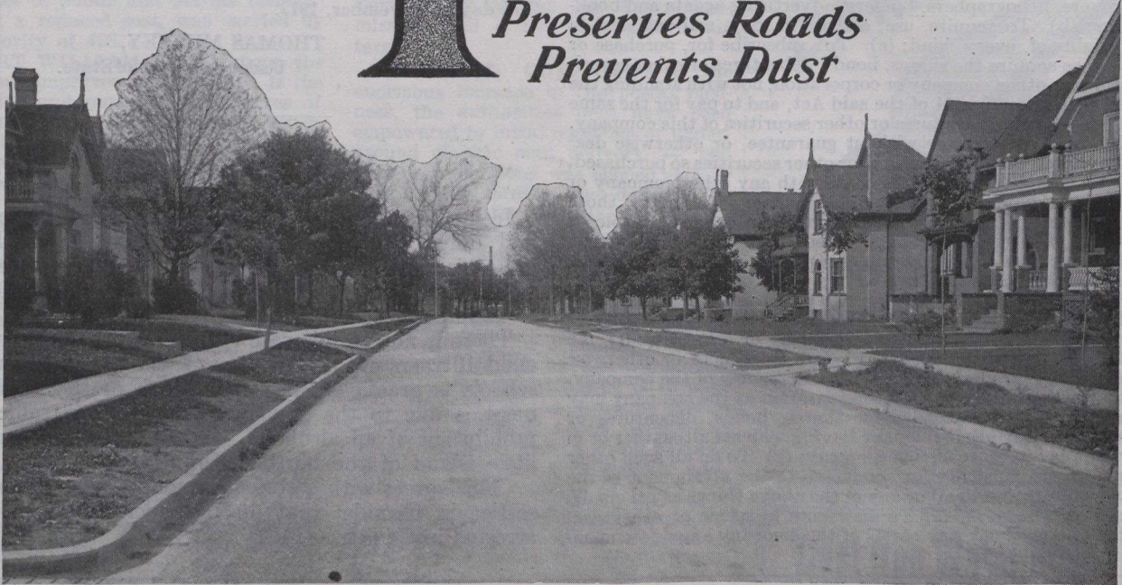
Foundry Street, Waterloo, Ont., Constructed with Tarvia Modern Pavement.
