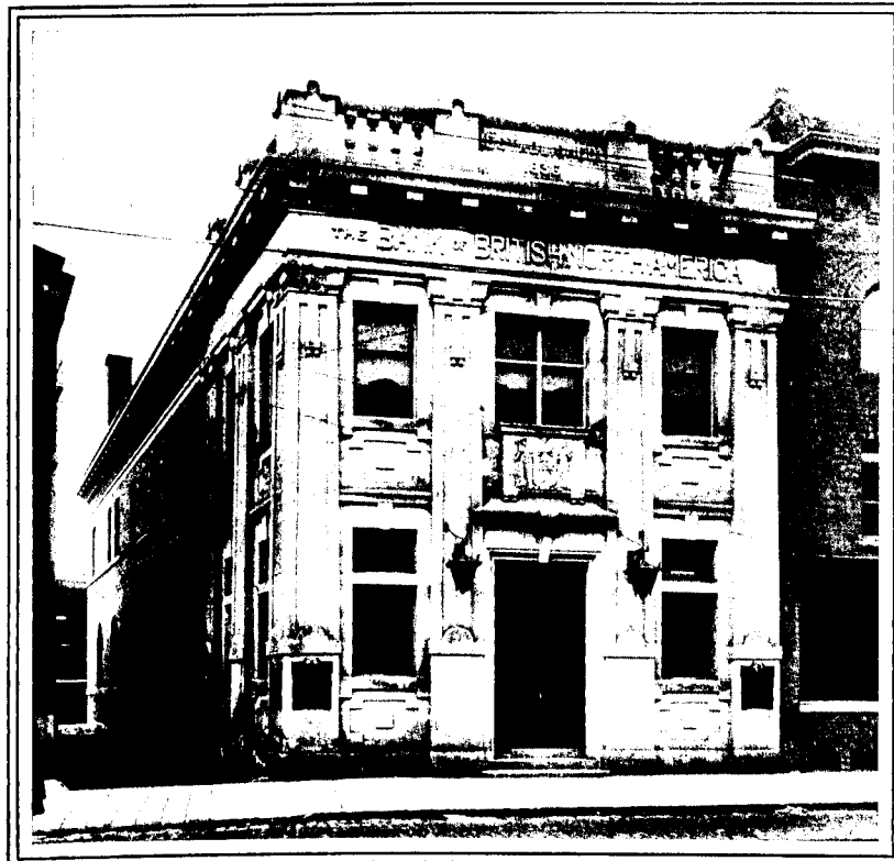
Bank of British North America, Toronto Junction Ellis & Connery, Architects, in which Milton Pressed Brick was used.
