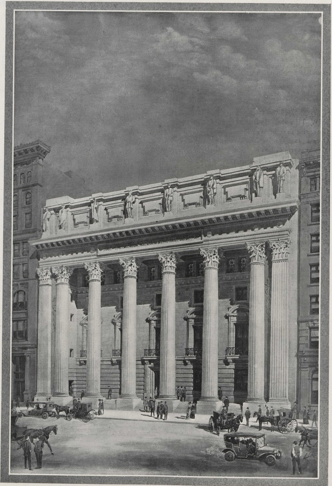
NEW BUILDING FOR THE CANADIAN BANK OF COMMERCE, NOW IN PROCESS OF CONSTRUCTION AT MONTREAL, SHOWING THE STRUCTURE AS IT WILL APPEAR WHEN COMPLETED. DARLING AND PEARSON, ARCHITECTS.
