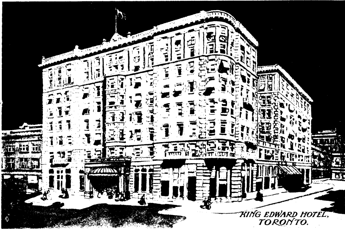
KING EDWARD HOTEL, TORONTO. FIREPROOFED THROUGHOUT WITH THE EXPANDED METAL SYSTEM OF FIREPROOFING.
