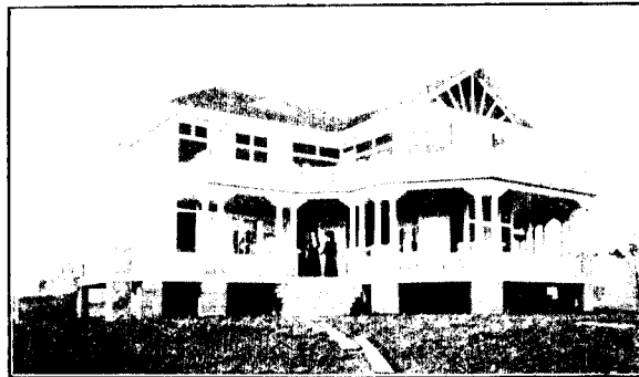
Waterloo County and Country Club House, Galt, Ont. Showing Cement Siding on "Herringbone" Lath, with half-timbered effect.
