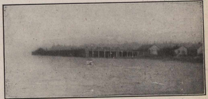
Port Mann Wharf, from the River.
