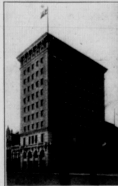
Union Bank Building, Winnipeg
