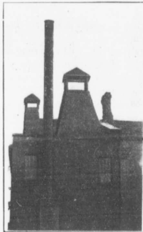
Fig. 5. Shewing view of roof of Steam Drier.
