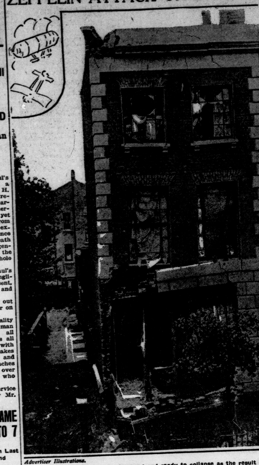
A house in London badly damaged and ready to collapse as the result of the first German air-raid on the metropolis. The bomb apparently landed on the front doorstep.
