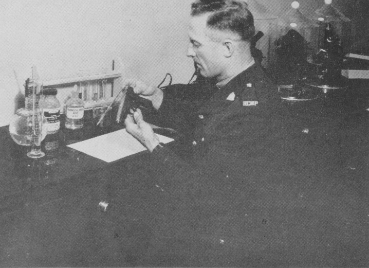
Crime Detection Laboratory technician restoring erased serial number on weapon.
