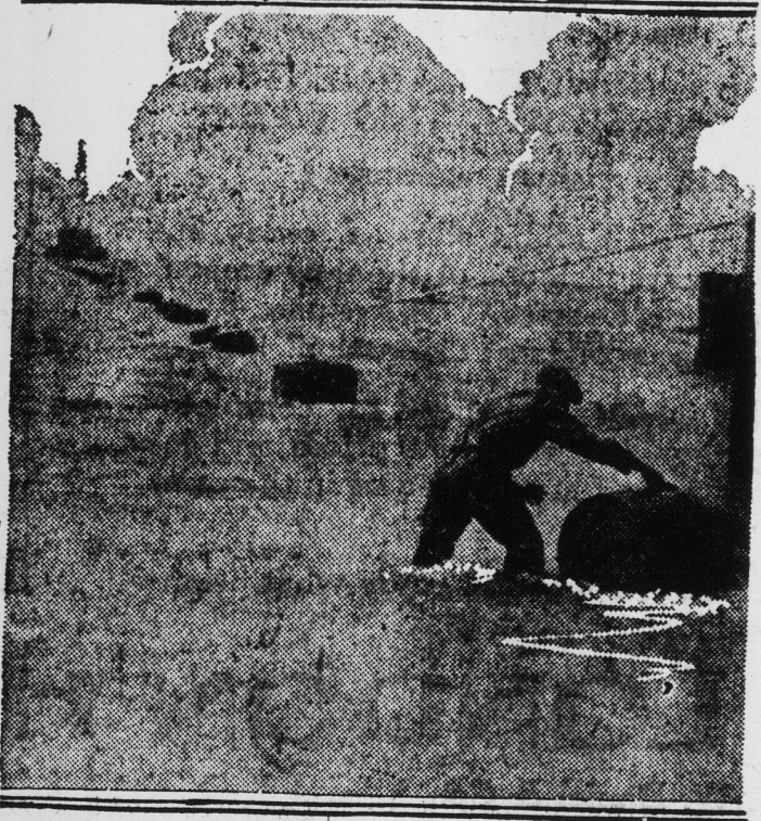
The nineteenth trans-Atlantic cable, and claimed to be the fastest of them all, is landed at Far Rockaway, Long Island. The eastern terminus of the cable is Penzance, England. The cable line is indicated by the series of black cables seen in the photo, the man at the shore guiding in the last few feet of the cable.
