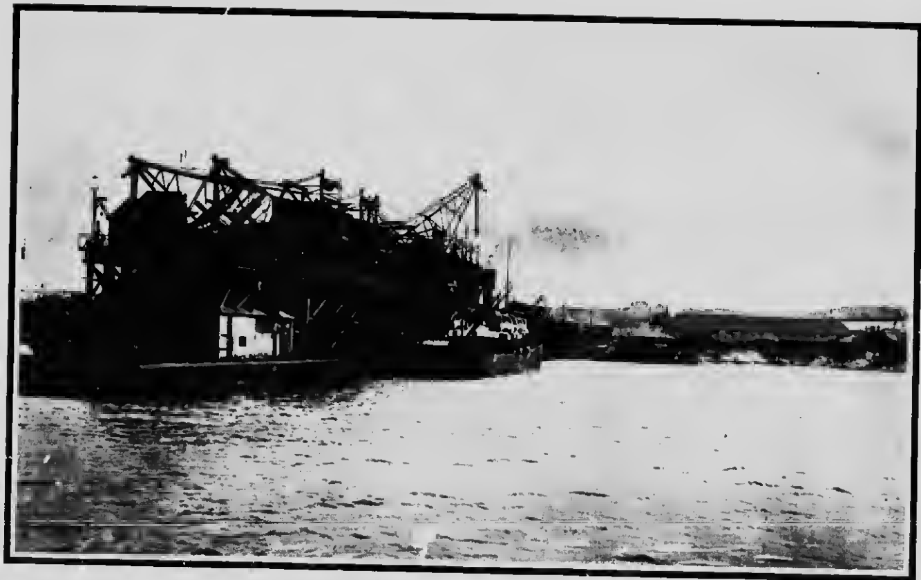
SHIPPING PIER, DOMINION IRON & STEEL COMPANY, SYDNEY.
