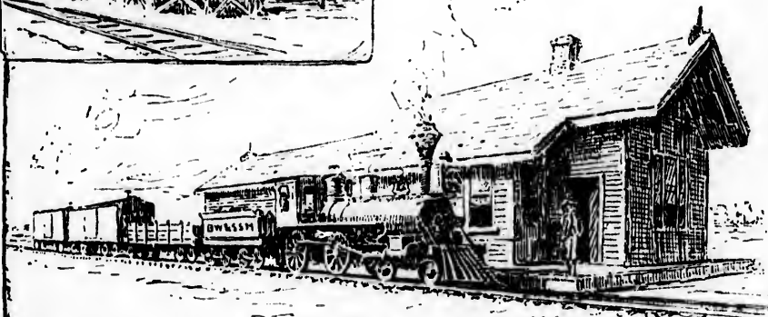
STATION AT VANDERBILT, AND WORK TRAIN —
