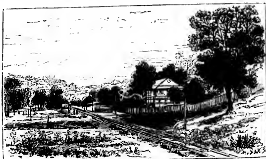
VIEW OF PARAISO, ON THE PANAMA RAILROAD.
