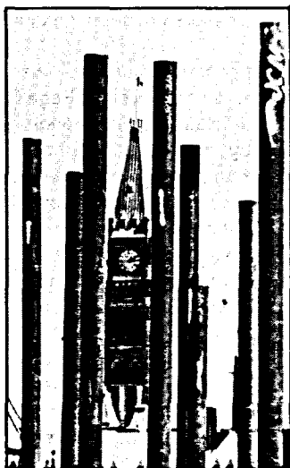
Steel pillars for the Museum of Man (under construction in Hull) frame the Peace Tower.
