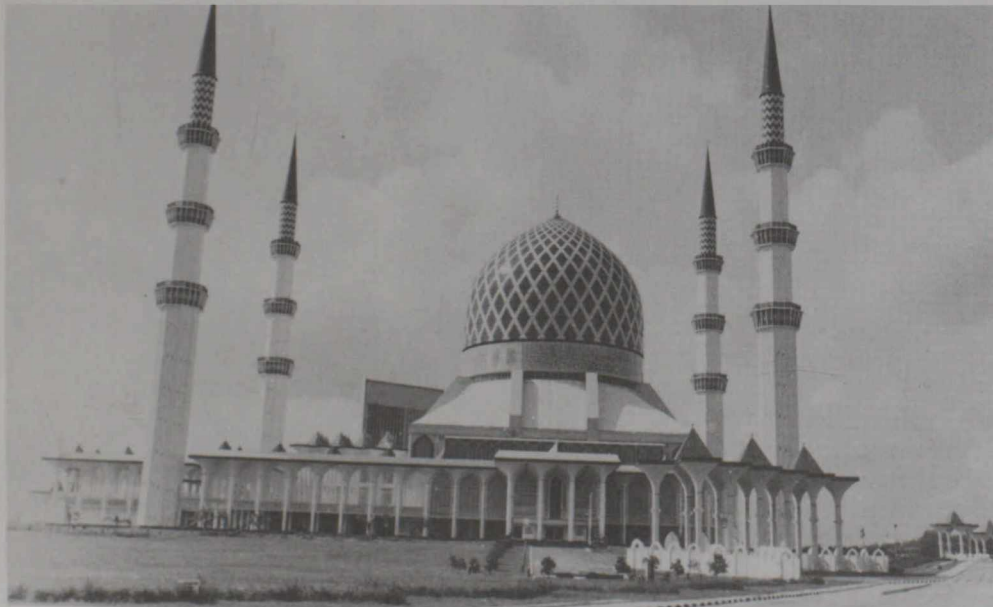
The attractive dome on the new Shah Alam Mosque was built using Canadian Triodetic technology.
