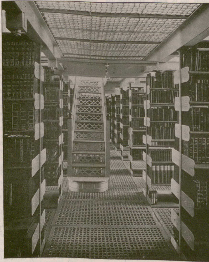
STACK ROOM, NEW LIBRARY, MCGILL COLLEGE, MONTREAL.
