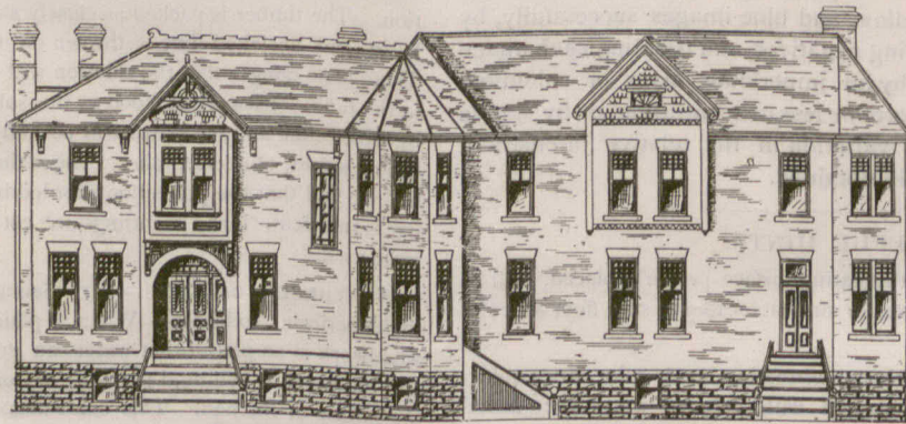
GENERAL AND MARINE HOSPITAL, COLLINGWOOD, ONT.
