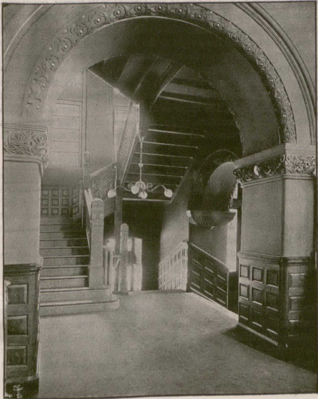
ENTRANCE HALL AND STAIRCASE, NEW LIBRARY, MCGILL COLLEGE, MONTREAL.
