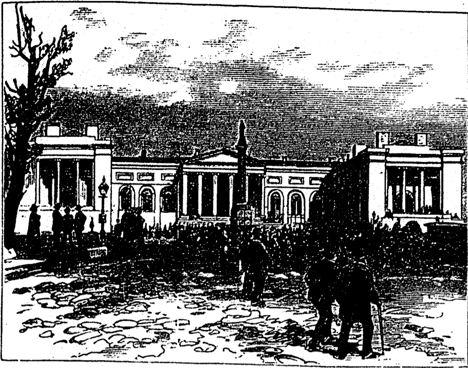
THE CITY HALL, WASHINGTON—COURT-ROOM ON THE RIGHT.
