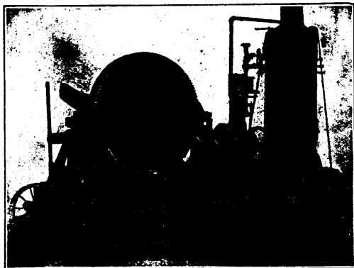
THE SMITH CONICAL CONCRETE MIXER ON TRUCKS COMPLETE WITH ENGINE AND BOILER.
