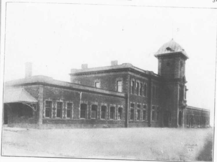
NEW INTERCOLONIAL RAILWAY STATION, TRURO, N. S.
