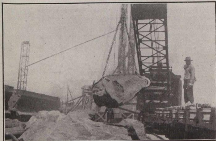
Fig. 6.—Handling "Plums" During Concreting
