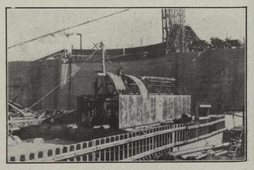
Fig. 4.—Lock 2 Breast Wall Under Construction and Forms Being Erected for Filling Tunnel in the West Lock Wall.
