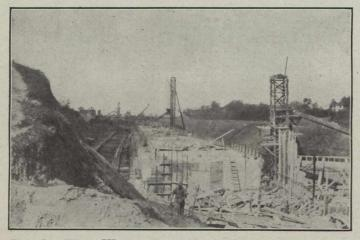
Fig. 2.-West Wall of Lock No. 1 Under Construction.
