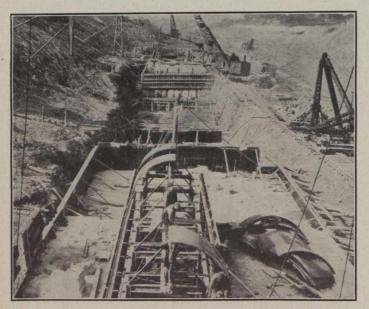
Fig. 3.—West Wall of Lock No. 2, Showing Erection of Steel Forms for Filling Tunnel.
