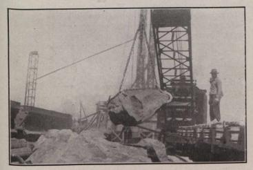
Fig. 6.—Handling "Plums" During Concreting
