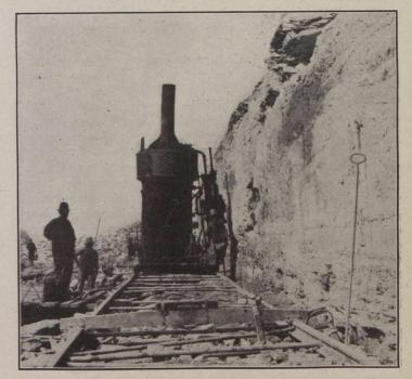
Fig. 7.-Rock Channelling Outfit at Work on Section 3.
