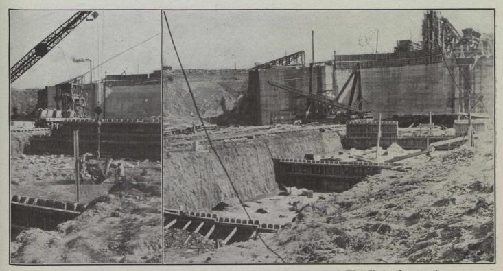
Fig. 5.-Views of Breast Wall of Lock No. 2, and Monoliths of West Lock Wall Under Construction.
