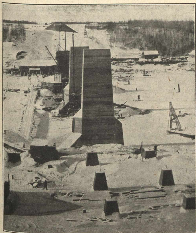
Piers Nos. 1 and 2, completed, Clover Bar Bridge, Alta.
