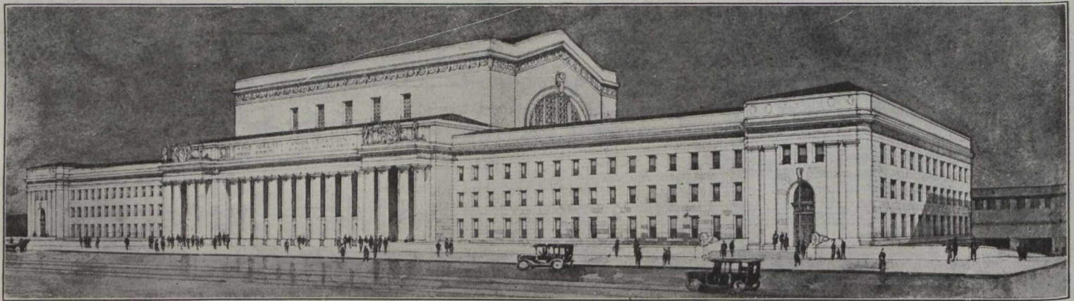
The new Union Station, Toronto, on which work has been started.
