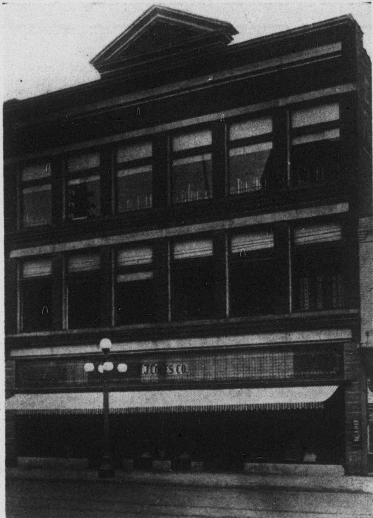
The fine exterior of the E. J. Coles Departmental Store, Woodstock, Ont.
