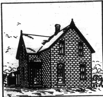
Concrete Residence of W. H. Fry, Fenwick, Ont. Size of Building, 28 x 32 x 18 feet high. BUILT WITH THOROLD CEMENT IN 1877.
