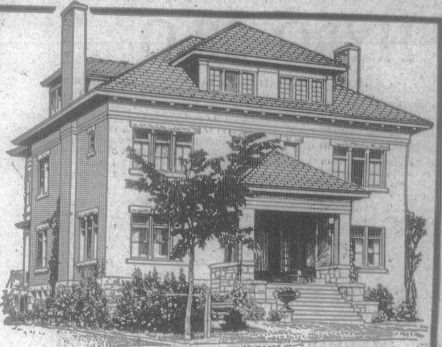
Home in Kingston roofed with Brantford Asphalt Slates
