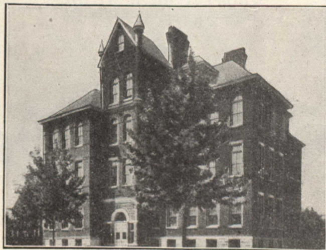
The Balaclava Street School, in which are the four Kelsey Generators that give such unbounded satisfaction to the Public School Trustees of St. Thomas, Ont.
