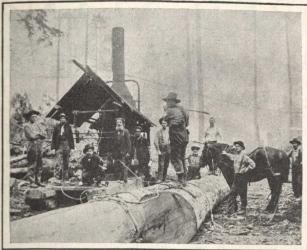
Drawing Saw Logs from the Bush to water's edge with a Steam Winch.
