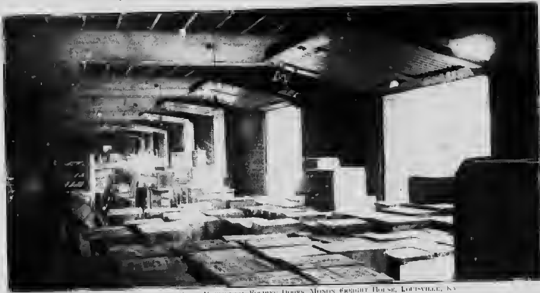
INSTALLATION OF 48 CROSS HORIZONTAL FOLDING DOORS, MONROE FREIGHT HOUSE, LOUISVILLE, KY. Doors are clear of floor, affording free space for the handling of goods.
