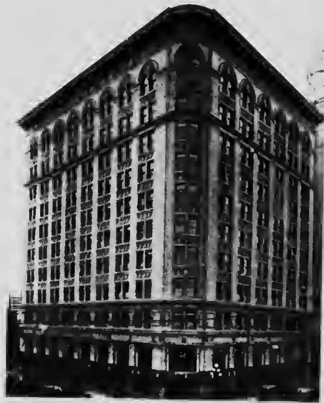
BIKES BUILDING, VANCOUVER, BRITISH COLUMBIA SOMERVELL & PETERSON, ARCHITECTS
