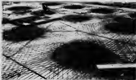
Reinforcing Steel in Place—"Mushroom System."
