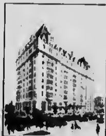
FORT GARRY HOTEL, WINNIPEG. ROOF SHEATHED WITH RU-BER-OID ROOFING. BASEMENT WATERPROOFED WITH IMPERVITE. ARCHITECTS—ROSS & McFARLANE.
