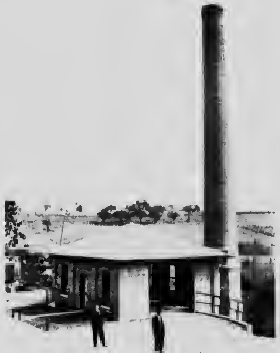
20 TON PLANT, NORTH BRADDOCK, PA.
