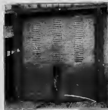
B. & O. ROUND HOUSE AT BALTIMORE, MD. Equipped with Wilson's Rolling Wood Doors, fitted with wire glass panels and wicket chocks.
