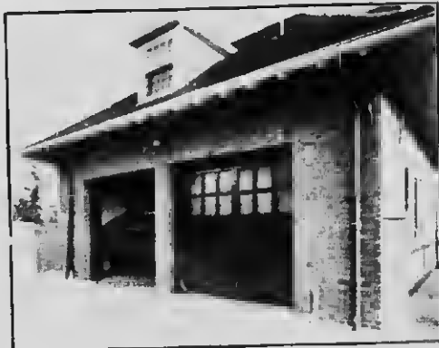
One door partially open, other closed. Glass in upper panel takes place of transom.
