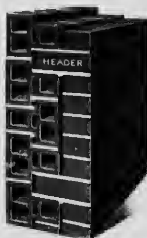
Wall of Denison Tile faced with Header of Common Brick
