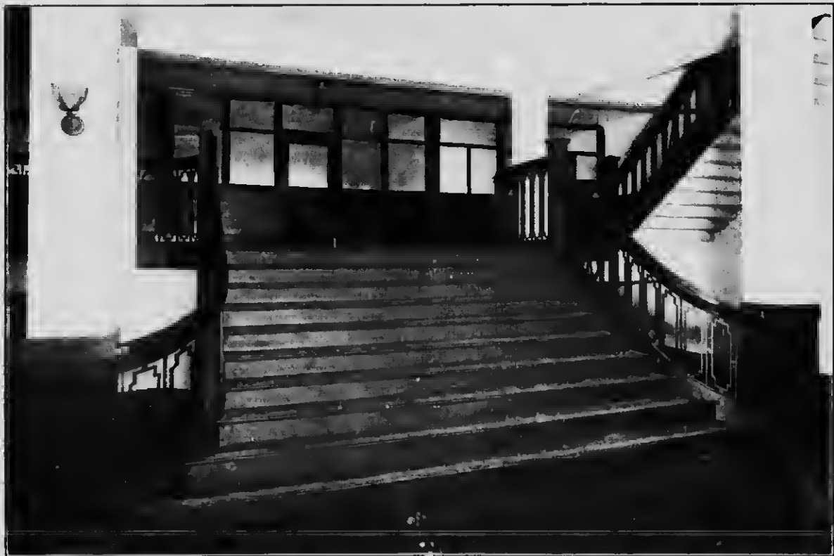
"MODERN METHOD" STAIRS, 16 FT. WIDE, INSTALLED IN THE DUKE OF CONSAUGHT SCHOOL, TORONTO. ONE OF THE FIFTY SCHOOLS IN TORONTO EQUIPPED WITH OUR STAIRS.
