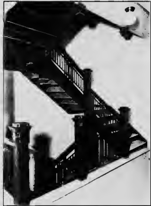
"MODERN METHOD" STAIRS, TORONTO GENERAL TRUSTS BUILDING
