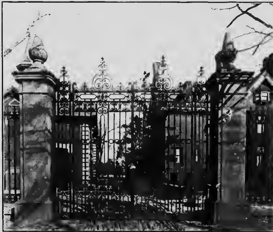
These gates, 15 ft. high and 13 ft. 7 in. wide, are part of a fence 700 ft. long and 12 ft. high, erected by us for the late Gen. Tuckett, of Hamilton — Stewart & Whitton, Architects, Hamilton
