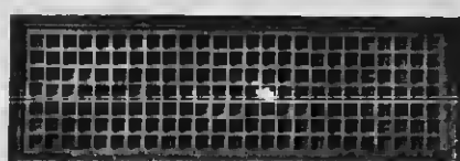
GRILLE HELD IN PLACE BY WOOD MOULINGS
