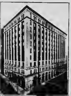
TRANSPORTATION BUILDING, MONTREAL Paristone Plaster was used exclusively in this building
