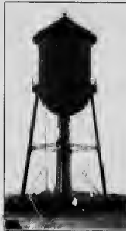
SPRINKLER TANK ON ROOF OF BUILDING. Capacity, 10,000 gallons. Height, 30 ft. to bottom.
