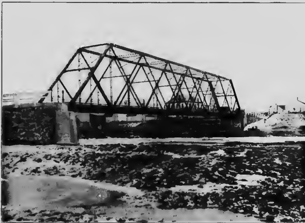
HIGHWAY BRIDGE, ST. EPIRO, LAKE ST. CHARLES COUNTY, QUEBEC. STEEL SPAN, FABRICATED AND ERECTED BY EASTERN CANADA STEEL & IRON WORKS, LIMITED.
