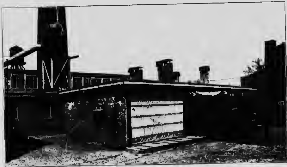
A CAR OF LUMBER ENTERING DRY KILN
