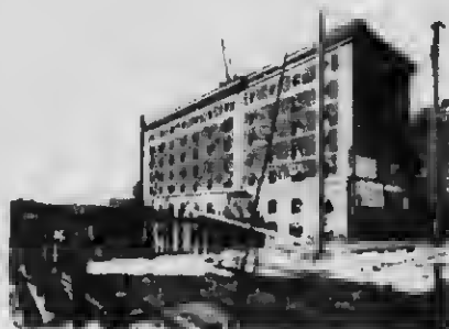
ROYAL ALEXANDRA HOTEL, C. P. R. W. D. Hammond, Church & Co., Engineers.
