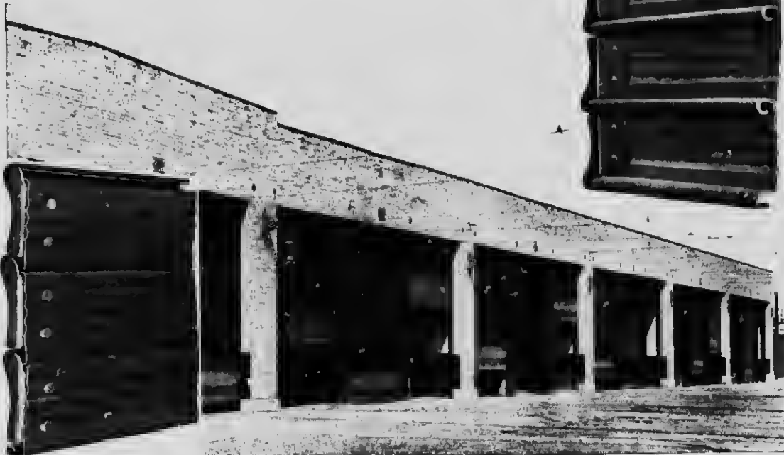
LINE OF ROLLING DOORS ON SINGLE STORY BUILDING. Total, 24 doors, each 12' 0" wide by 18' 0" high.
