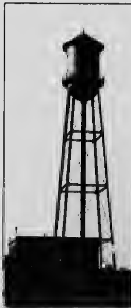
SPRINKLER SYSTEM, GOLDIE & McCLELLICH C. CO., LTD. Capacity, 10,000 gallons. Height, 88 ft. 6 in. to bottom.
