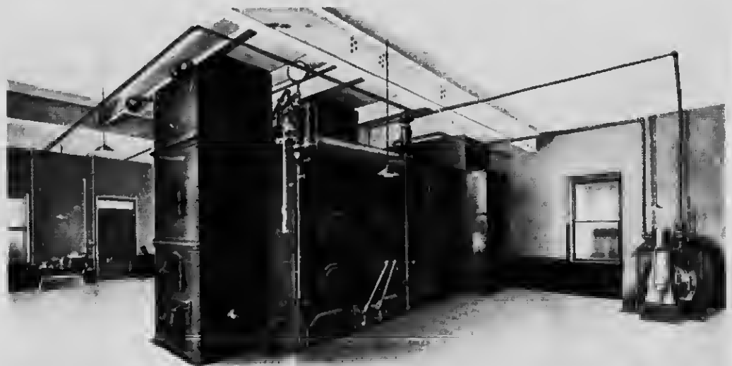
INTERIOR VIRGINIA, MINN., 25 TON PLANT
