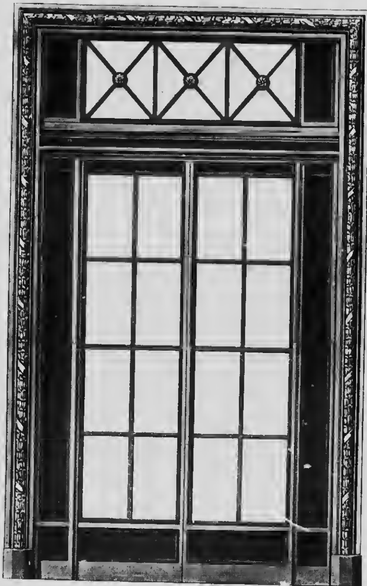
ELEVATOR ENCLOSURE. A. E. REA BUILDING, OTTAWA. ROSS & McDONALD, Architects
