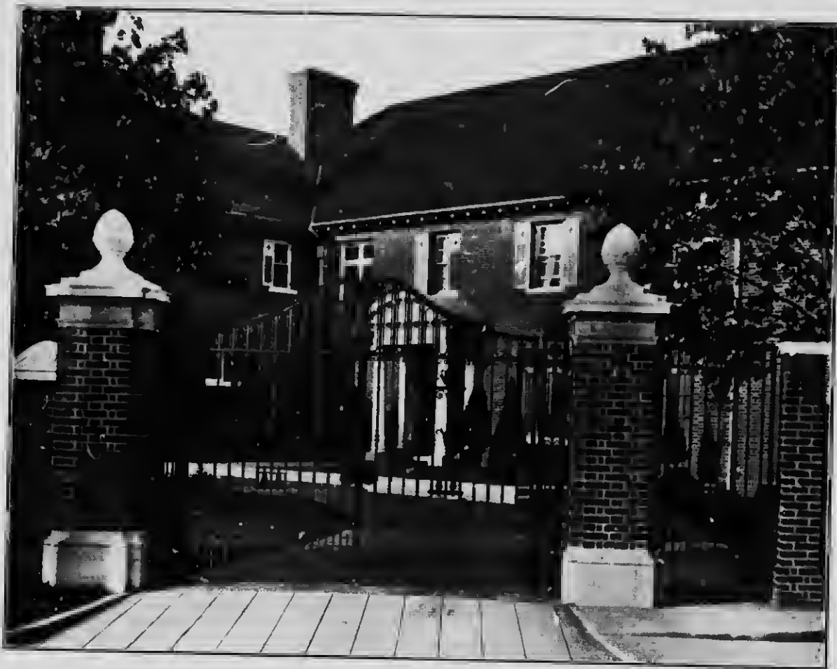
RESIDENCE, GERRARD B. STRATHY, TORONTO. Eustace G. Bird, Architect
