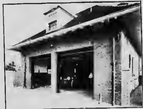
Doors fully opened, and ready, though Automobile is near. No valuable space is occupied either opened or closed.
