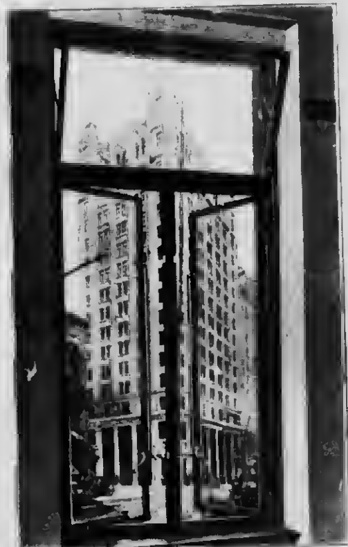
CANADIAN PACIFIC RAILWAY OFFICE BUILDING, TORONTO. CRITTALL "UNIVERSAL" CASEMENTS INSTALLED THROUGHOUT. DESIGNED BY PEARSON, MOHR & CO. ARCHT. & ENGINEERS LTD. TORONTO.
