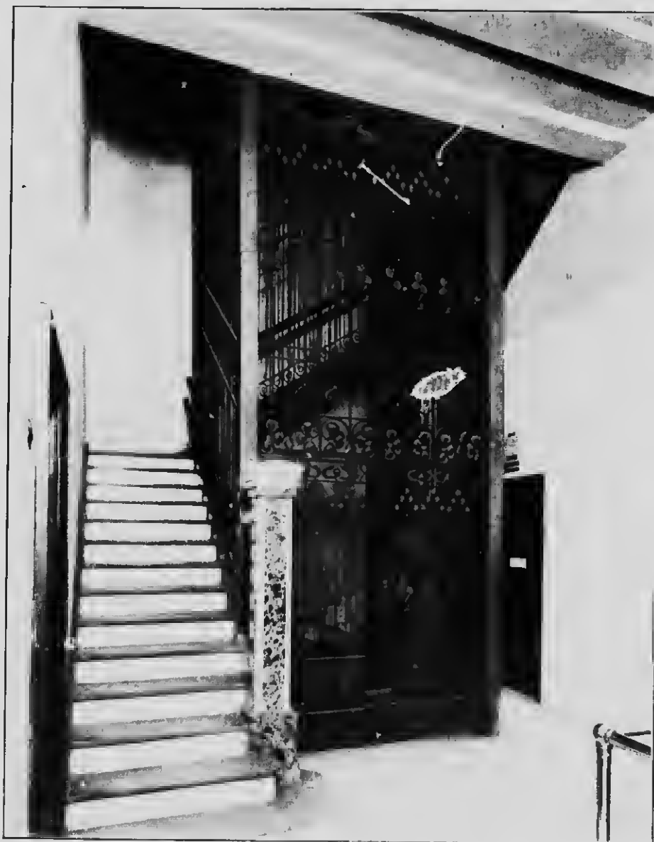
"MODERN METHOD" STAIRS AND ELEVATOR ENCLOSURE, WORLD BUILDING, TORONTO
