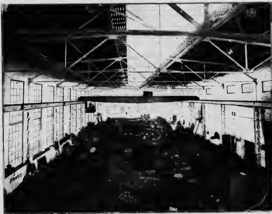
INTERIOR OF OUR NINE FOUNDRY - CAPACITY, 25 TO 30 TONS DAILY
