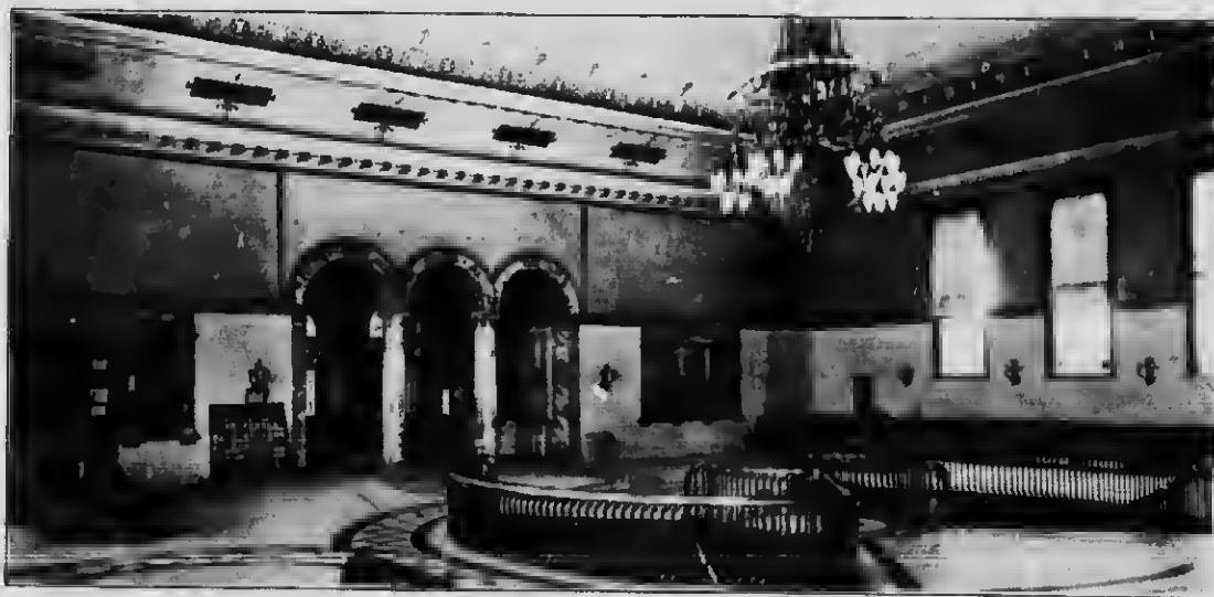
CHICAGO, BURLINGTON AND QUINCY RAILROAD STATION, OMAHA, NEBRASKA Showing Hy-namel brick which has been in use more than sixteen years, and has no trace of cracking, scaling or discolouring.
