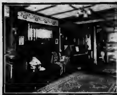
LIVING ROOM WITH BEAVER BOARD WALLS AND CEILING.
