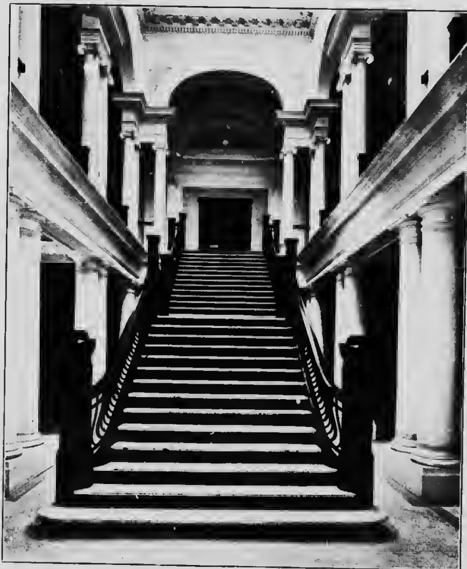
"MODERN METHOD" STAIRS, MARBLE TREADS, INSTALLED IN THE NEW COURT HOUSE, EDMONTON.
