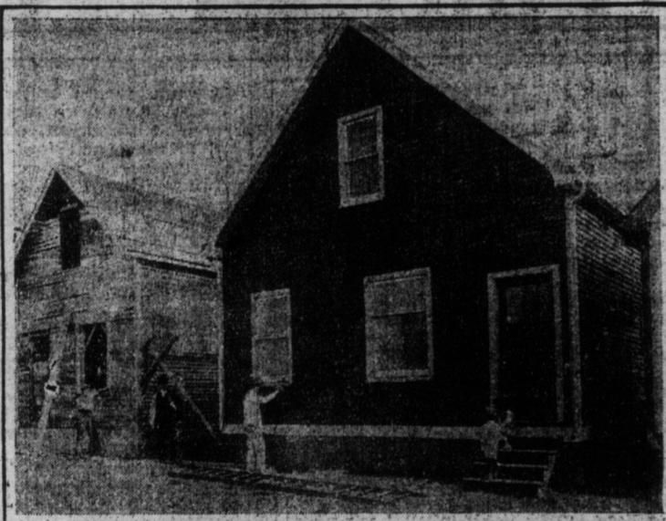
This shows a couple of the cottages in the process of erection and finishing. They are well constructed of Manitoba siding, tar paper lining, good heavy board siding and plastered inside; four rooms, all nicely arranged.
