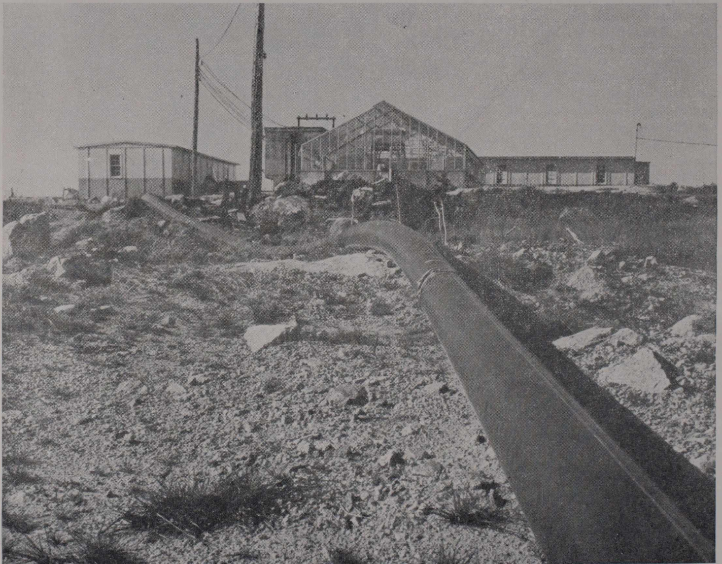
The seaweed research station at Fink Cove. The pipe in the foreground carries seawater to the station.
