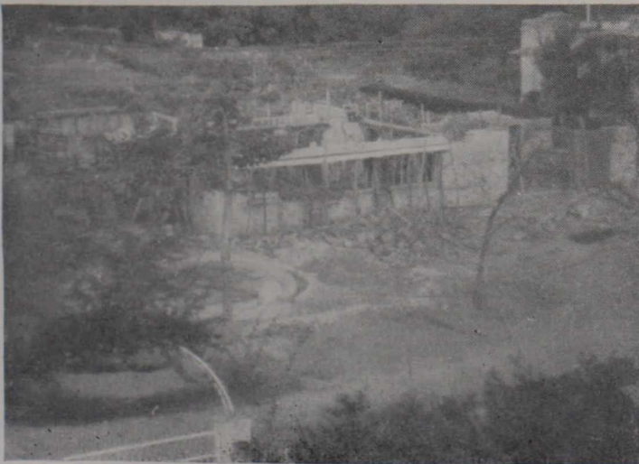
Adult Education Building under construction at Seva Mandir, Udaipur.
