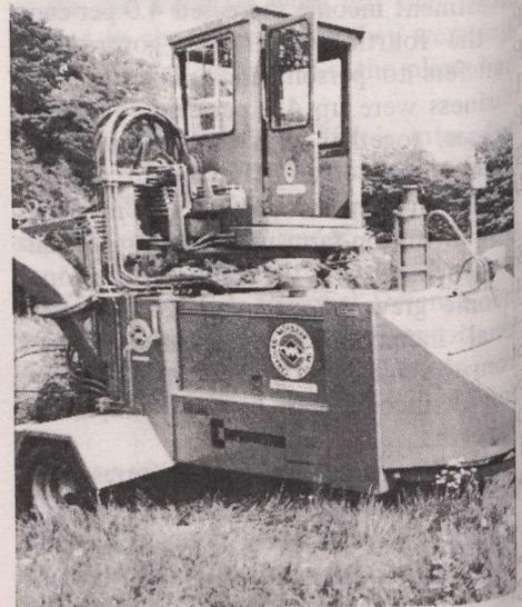
*The Total Chiparvestor, a new product of Morbark Industries, Inc. of North Bay, Ontario, transforms in minutes twisted undergrowth and trees normally allowed to decay, into fuel chips, which are later converted to energy by a wood-burning boiler system. A ton of green wood is about equal to 6,500 cubic feet of natural gas, a third of a ton of coal or one barrel of oil.*
