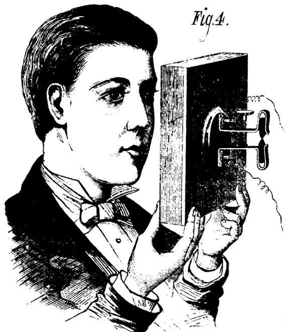
Fig. 4.—MICRO-TELEPHONE USED AS A TELEPHONE.
