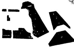
Fig. 13. - View of the Separate Pieces of the Plow Body, minus the Mould Board.
