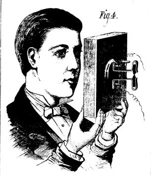
Fig. 4.-MICRO-TELEPHONE USED AS A TELEPHONE.
