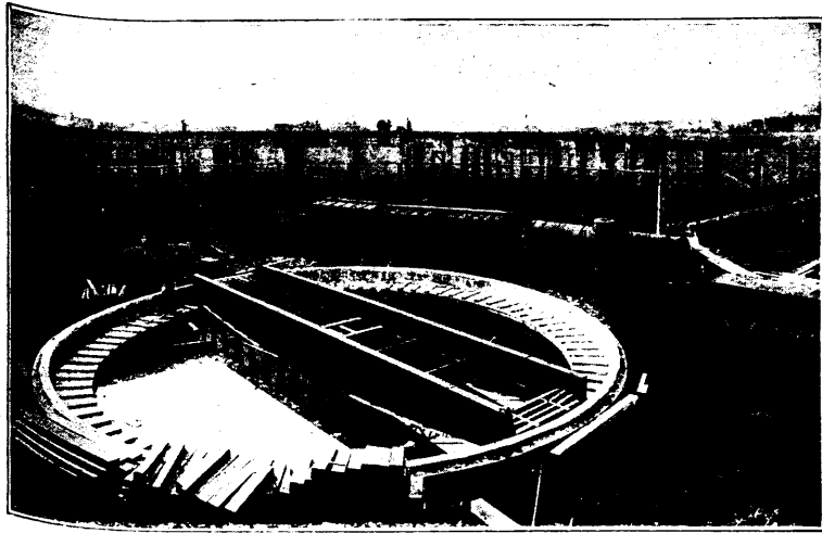
SHOWING G.T.R. ROUND HOUSE AT MIMICO, ONT., IN PROCESS OF CONSTRUCTION.
