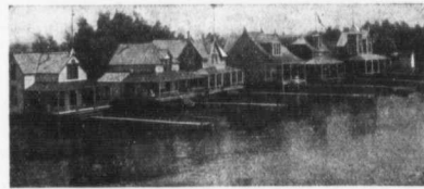
COTTAGES AT THE FLATS.
