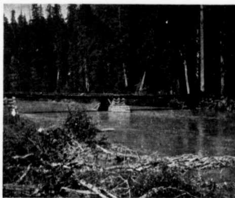
Fish River Bridge, at Goldfields.
