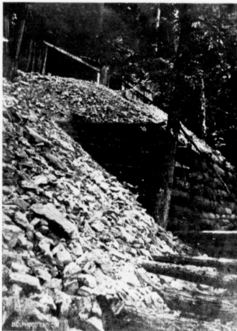
Ore Dump, No. 6 Tunnel Eva Mine.
