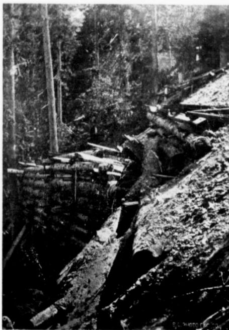
Ore Dump, No. 3 Tunnel, Eva Mine.
