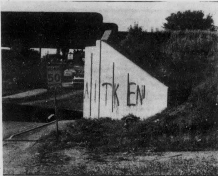
Underpass hit by Aitken painters
