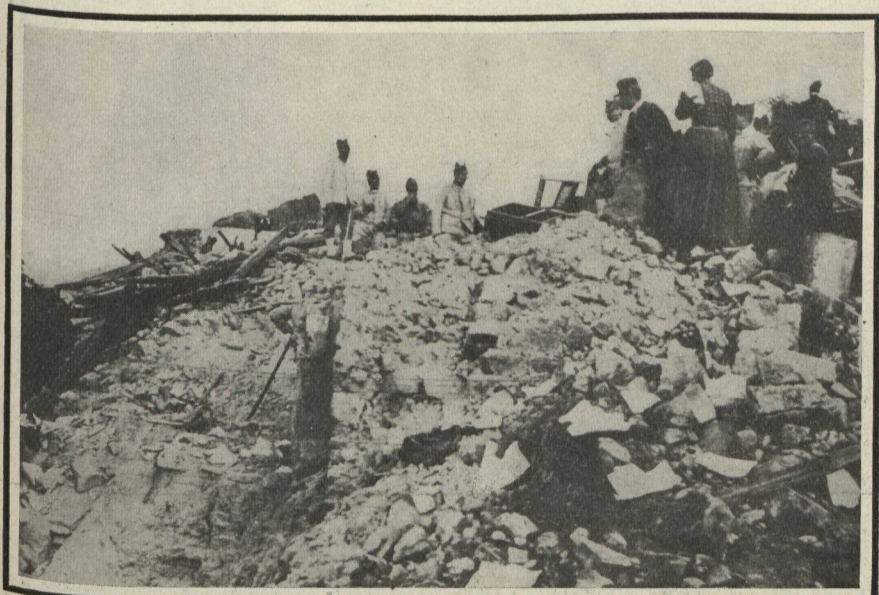
Ruined Houses in Calabria with Soldiers doing salvage work.
