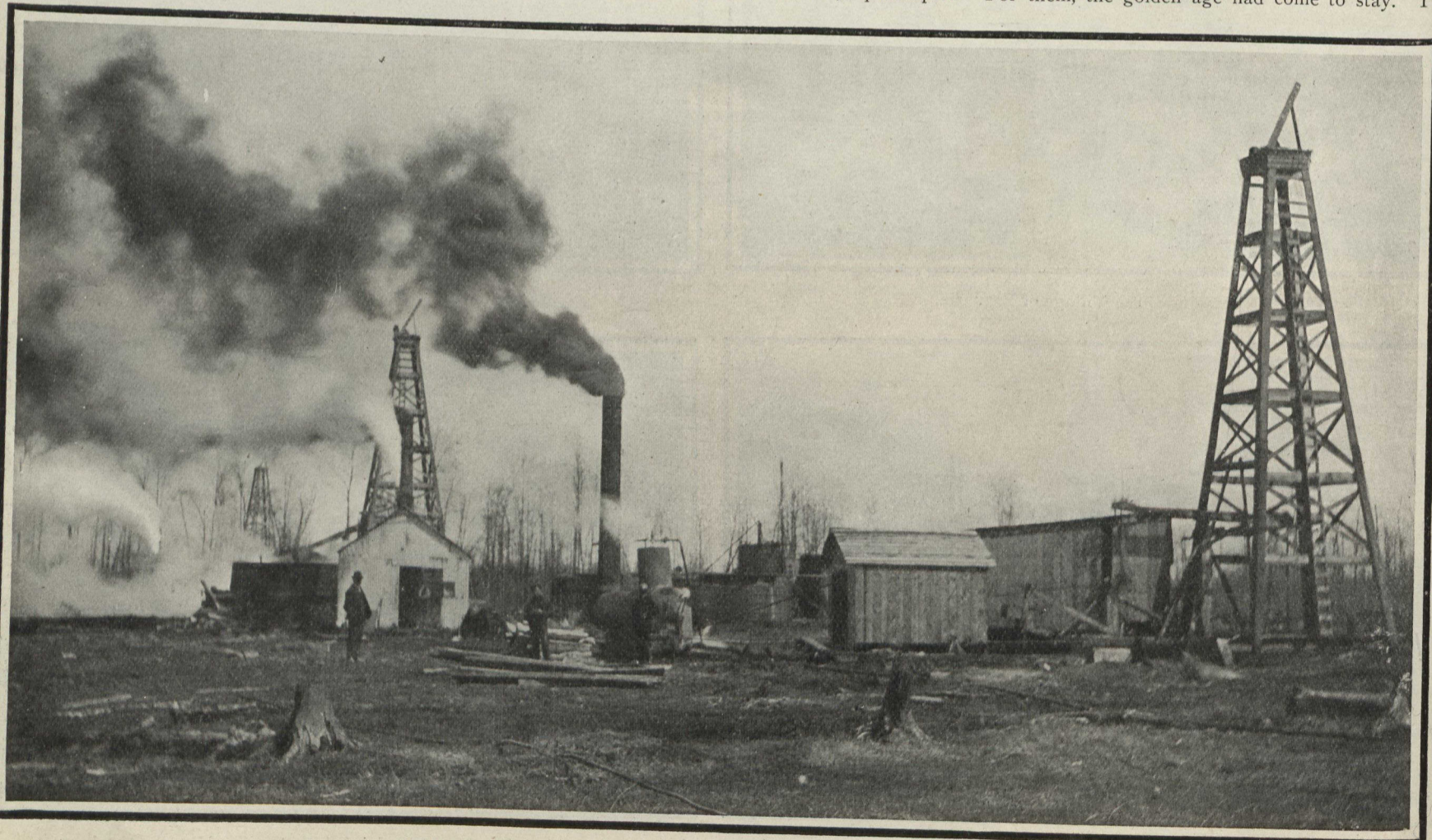
Early operations in the Tilbury Field. Showing Tool-house on the left.
