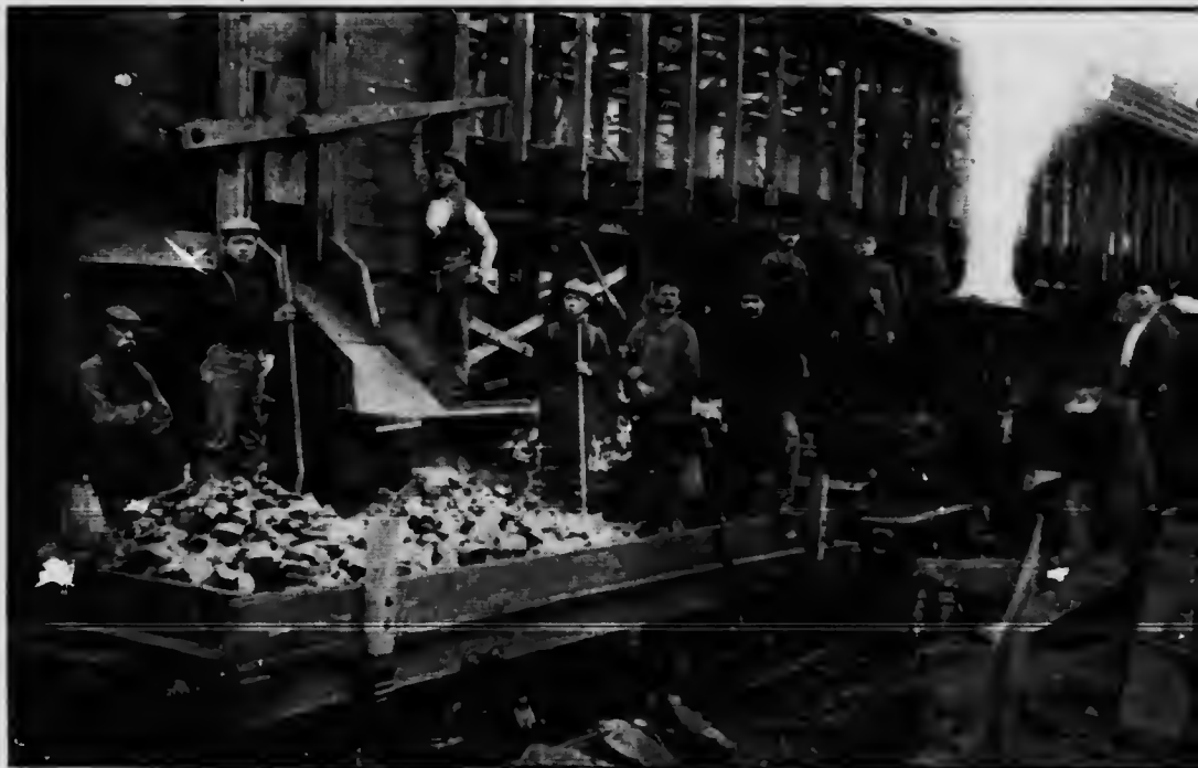
LENORA NEW SORTING SHED AND ORE BUNKERS.
