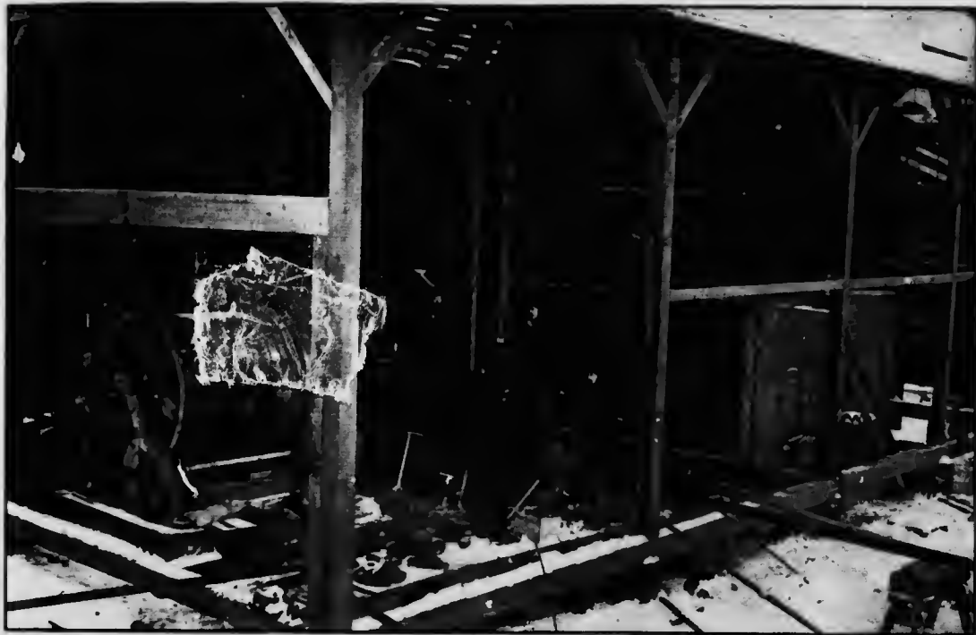
TYEE HOIST AND COMPRESSOR PLANT.
