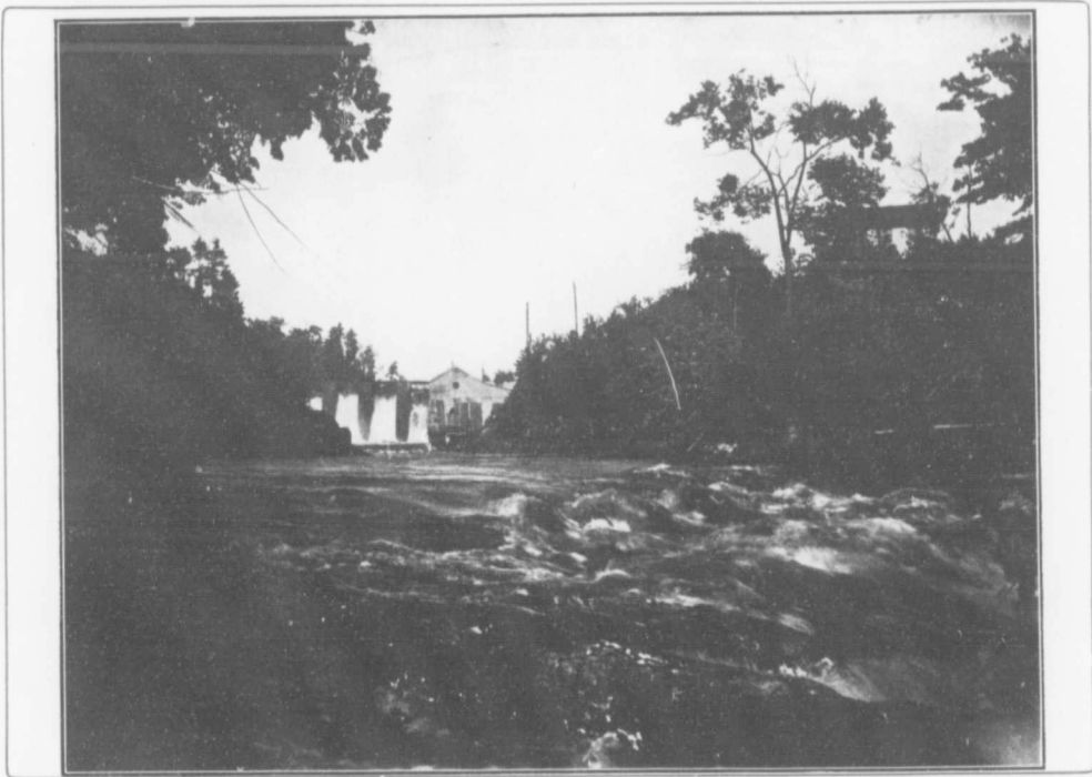
RAGGED RAPIDS ON SEVERN RIVER, THE SOURCE OF ORILLIA'S ELECTRIC POWER
