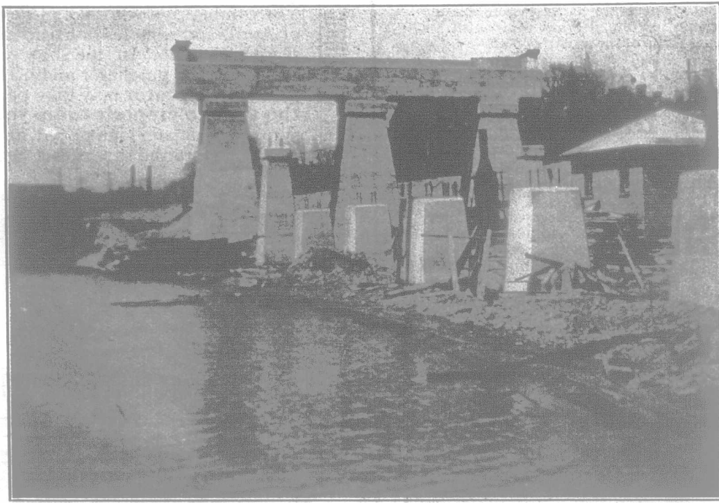
Concrete piers recently completed for bridge over railroad at Sunnyside, Toronto, Ont. Crushed stone and cement supplied by Alfred Rogers, Limited.
