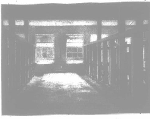
Cow Stable at Central Experimental Farm, Ottawa. Showing feed passage, mangers, drinking fountains, and control tank at end of
