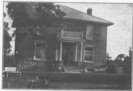
Fine Cement Farm Home, Owned by Mr. R. W. Walker
