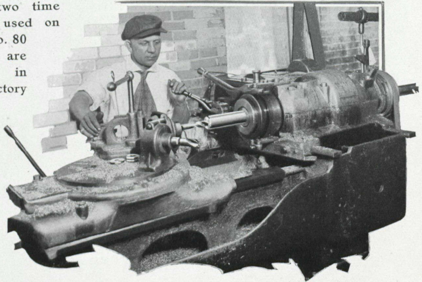
BORING AND CUTTING OFF TIME RINGS
