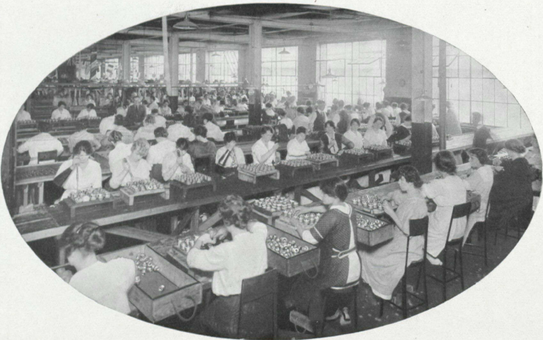
GENERAL VIEW OF ASSEMBLING ROOM
