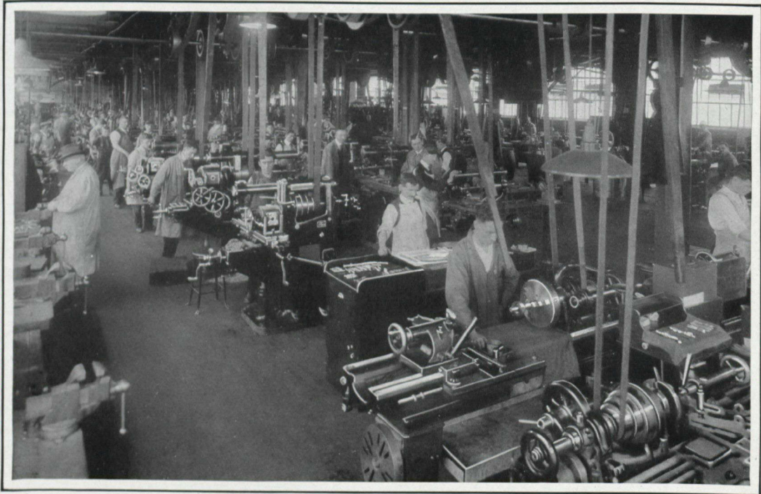
GENERAL VIEW TOOL ROOM
