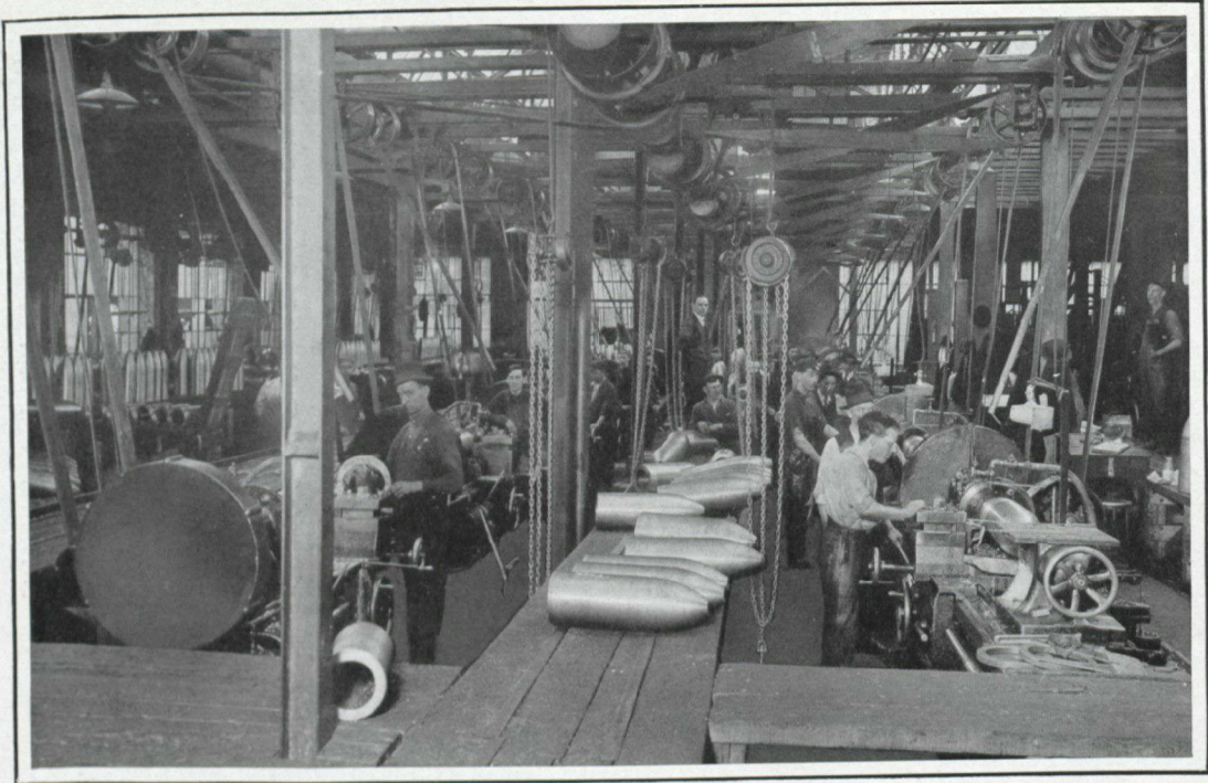
GENERAL VIEW FINISHING TURNING
