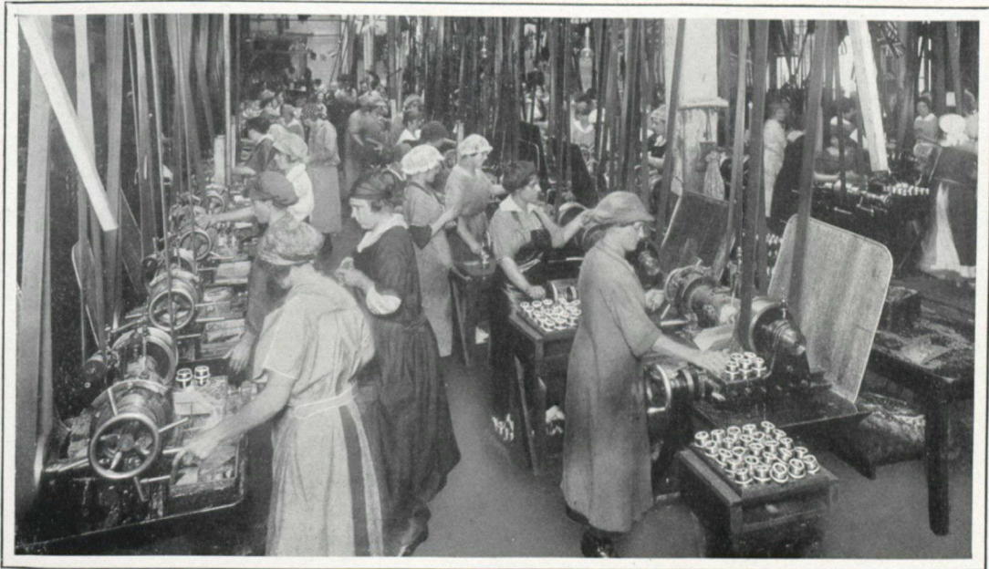
GENERAL VIEW OF THREAD MILLING DEPARTMENT
