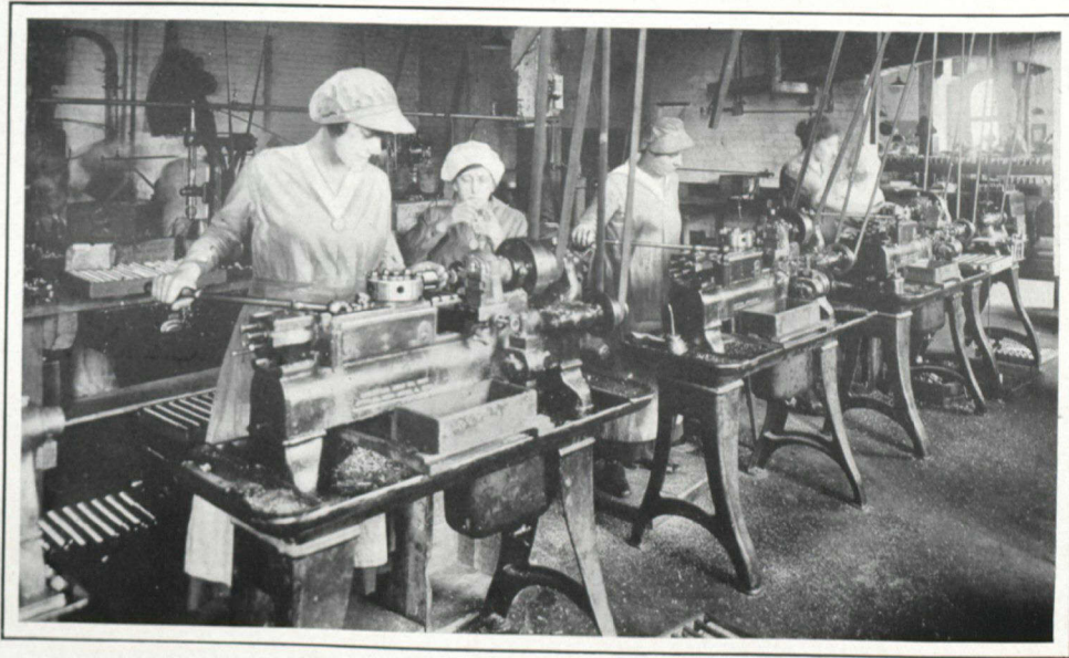
MACHINING BASE PLUGS
