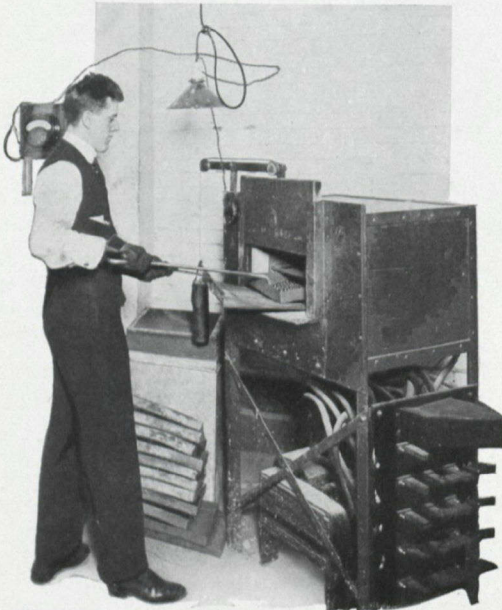
HEAT TREATMENT OF FERRULES FOR ARMING
