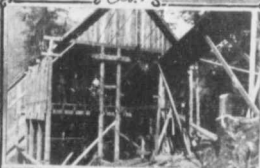
LOWER TRAM TERMINAL ORE BINS
