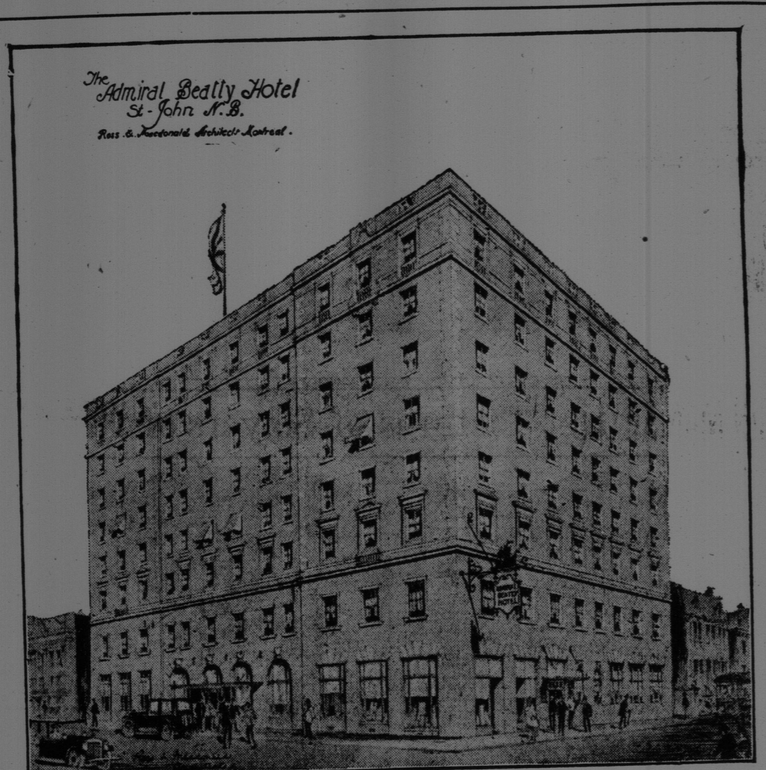
Here is the Admiral Beatty, the big new hotel, work on which was commenced today on the site of the old Dufferin Hotel, King Square. The signing of the contract today followed a campaign of less than a week during which a Citizen's Committee raised in subscriptions $121,350, of which $120,300 was needed before the project was assured. Many people today witnessed the start of actual construction work.
