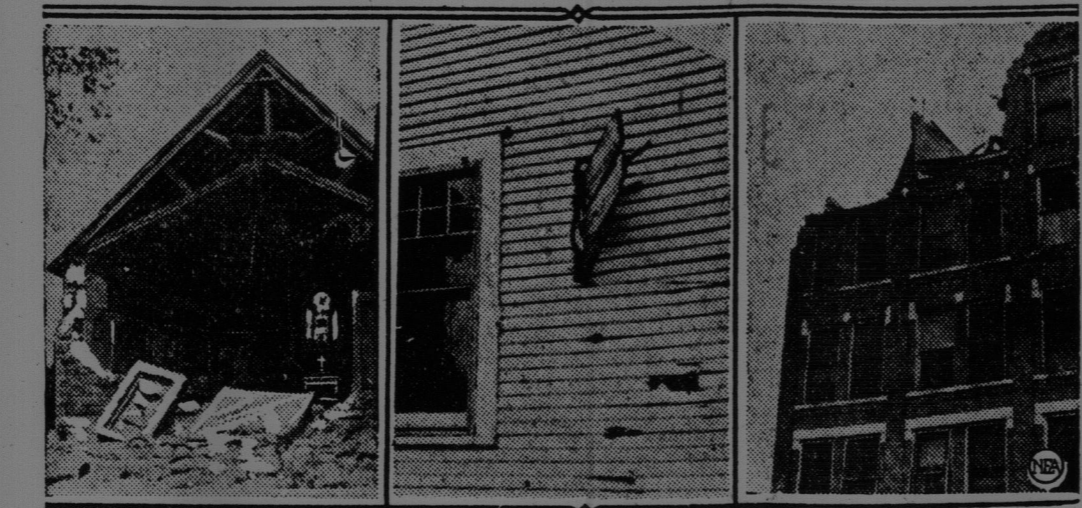
These are just a few of the freakish stunts a tornado pulled in Algona, Kas. The picture at the left shows the Episcopal Church minus its front. In the centre one sees a load, from some other building, driven into the side of a house. At the right is seen a five-story office and apartment building with one corner entirely gone.
