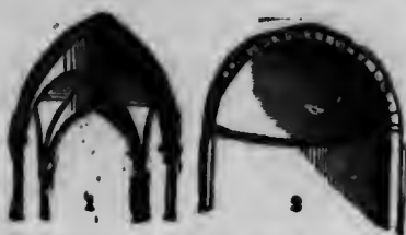
1, Gothic Groined Vault. 2, Spherical or Domical Vault.
